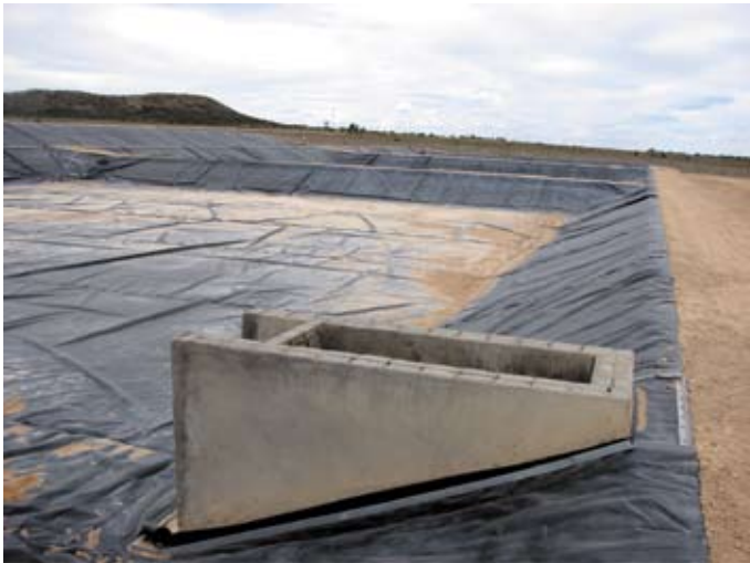
Upgrading of existing oxidation ponds
