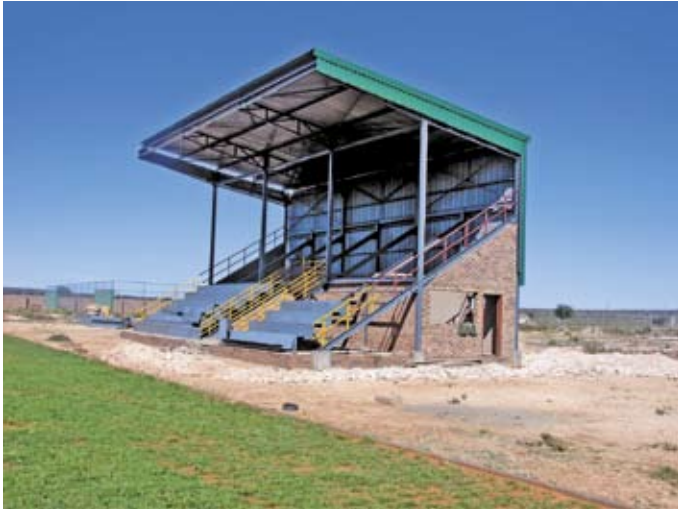
Hopetown – Pavilion under construction of sports field
