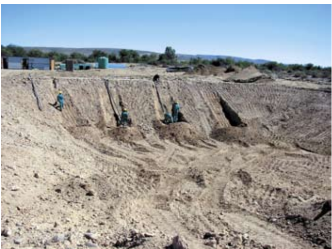
Workers busy sloping embankments
