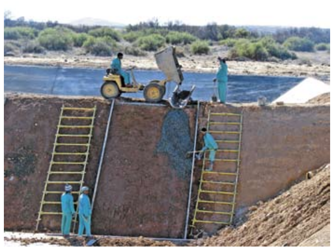
Excavations of primary ponds
