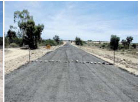
Primed base course ready to be sealed
